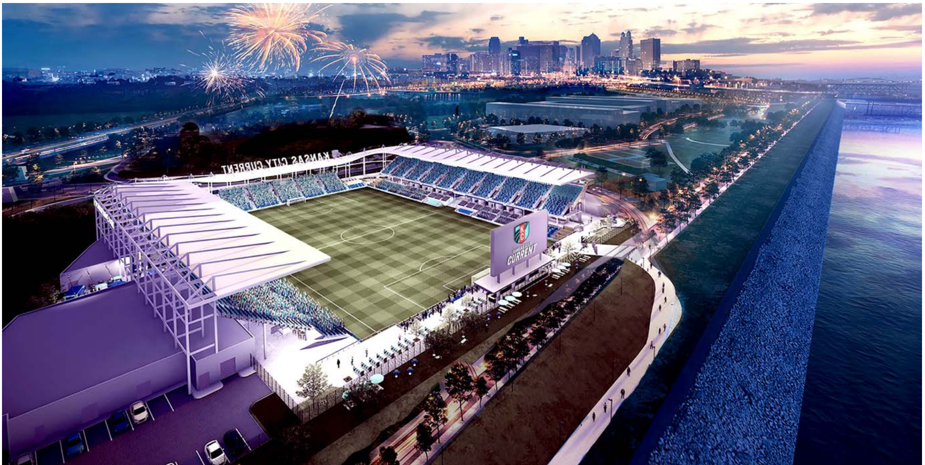
KC Current Stadium At Berkley Riverfront Park
